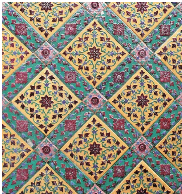
Figure 1-8: Bencharong tiles covering a wall at Wat Ratchabophit, Bangkok. Photo by author, 2017.
